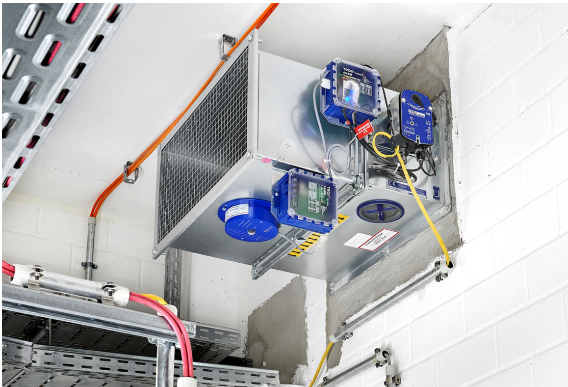
©TROX: Fire damper of the FK-EU series as a flow duct with smoke detector integrated into the TROXNETCOM system
