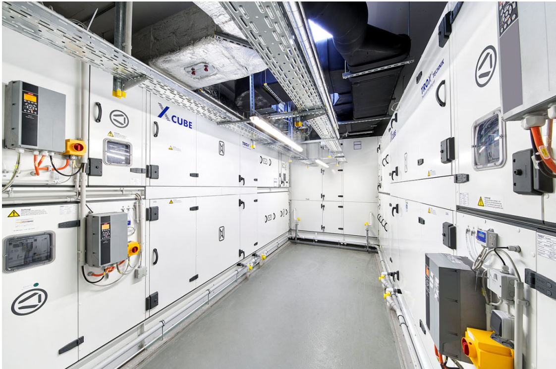
©TROX: X-CUBE housing used as an insulated ventilation duct
